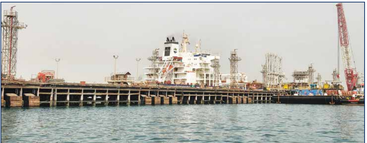
Marine Maintenance Works at MAA Refinery
