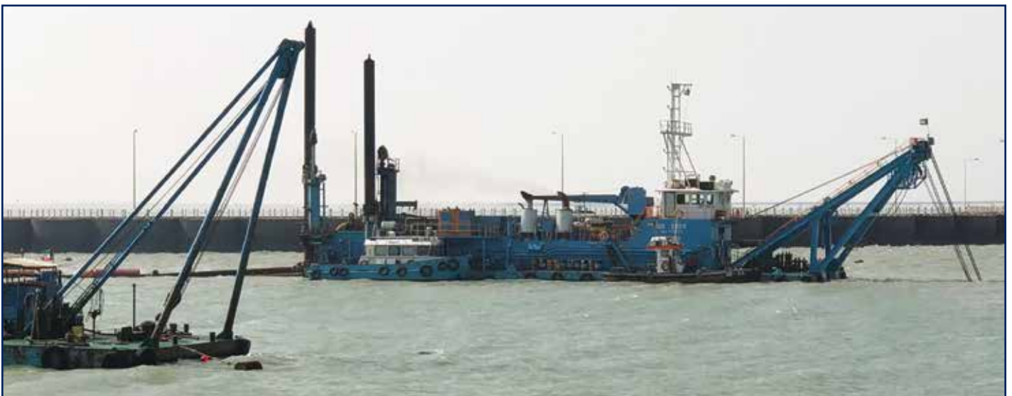
Maintenance Dredging of Seawater Intake Channel at Subiya Power & Water Distillation Station
