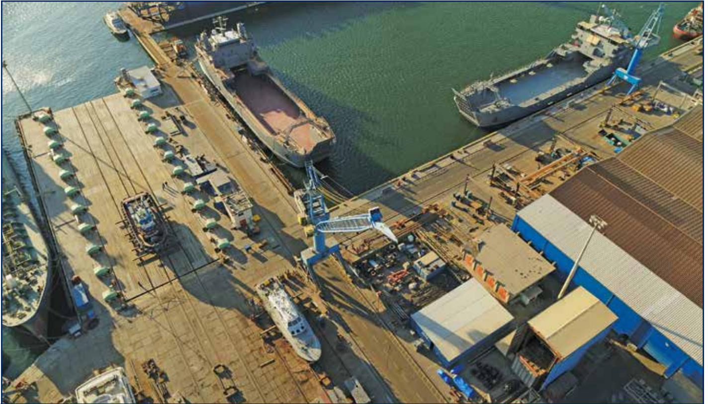
Aerial Overview of Syncrolift & Jetties
