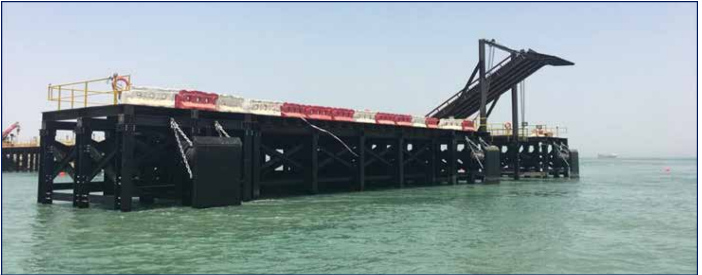
Construction of Offloading Jetty at Ras Al - Ard Logistics Station
