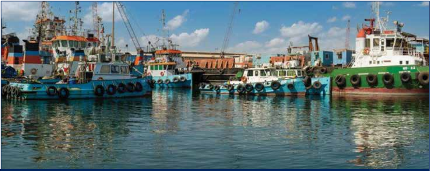
Berthing Facilities at Shuwaikh Port, Kuwait
