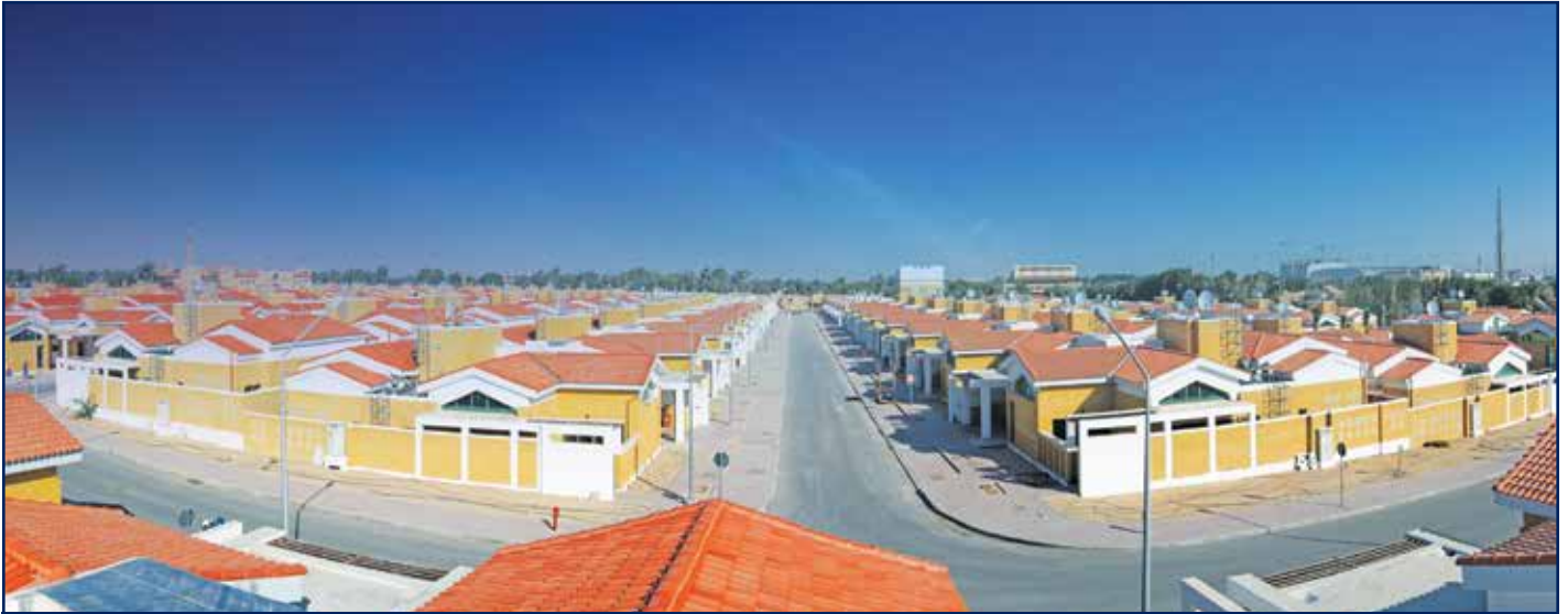
Construction, Completion and Maintenance of 160 New Houses in South Ahmadi Area
