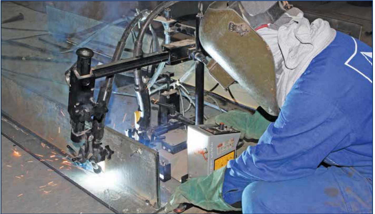
Welding of T-Plate Stiffener Using Auto-flux Core Arc Welding Machine
