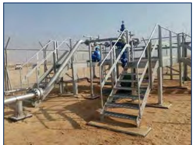
Construction of Flowlines and Associated Works in West Kuwait Area 2
