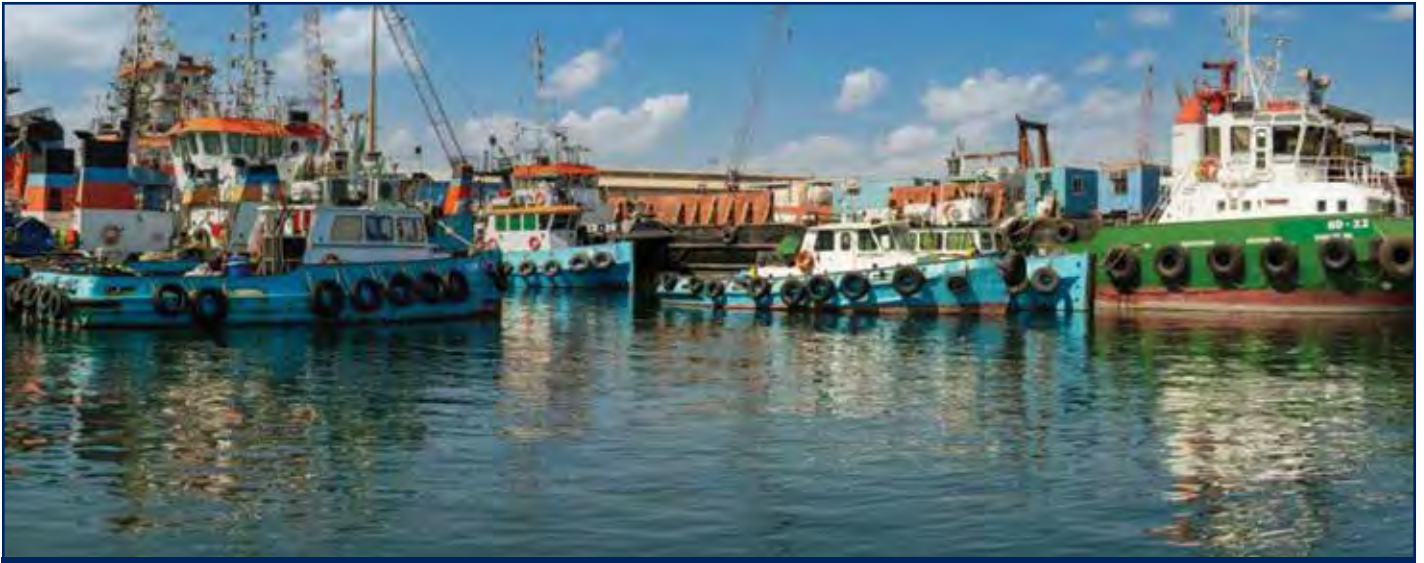
Berthing Facilities at Shuwaikh Port, Kuwait
