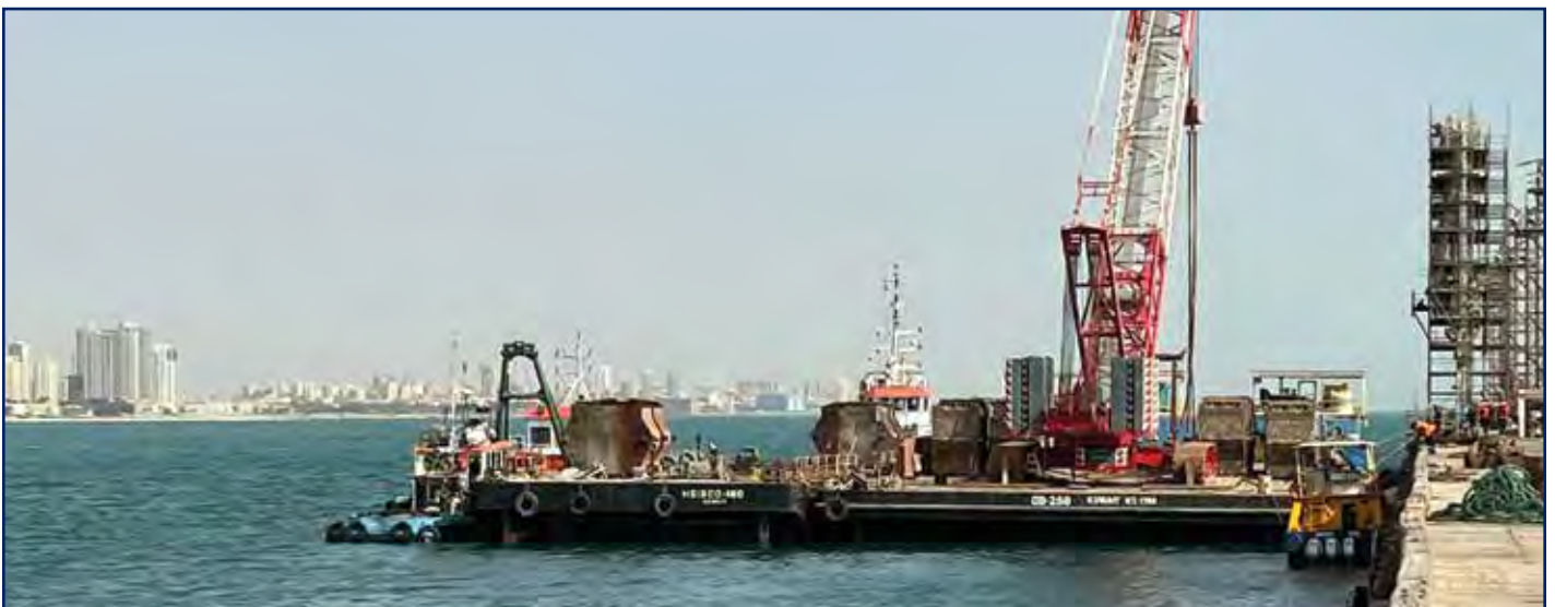
Heavy Equipment Barge for Marine Maintenance Works at Mina Al Ahmadi Refinery
