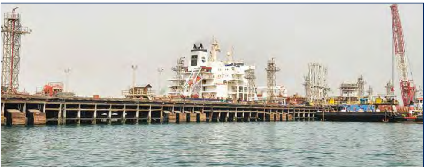
Marine Maintenance Works at MAA Refinery
