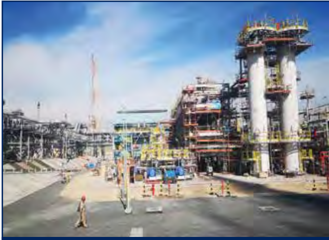
Structural, Mechanical, Piping, Electrical and Instrumentation Works for Sulphur Area at Az-Zour Refinery project - EPC Package 2&3
