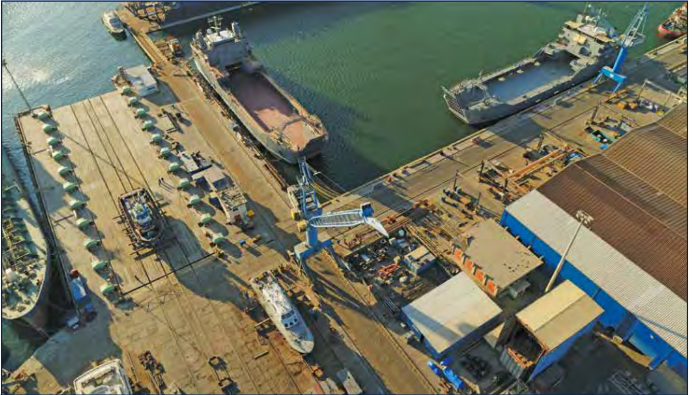
Aerial Overview of Syncrolift & Jetties
