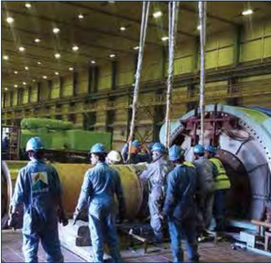
Generator Maintenance Works - MEW Az-Zour Power Station
