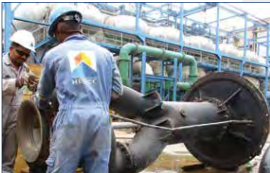
Maintenance of Blowdown pump - Shuaiba South Power Station
