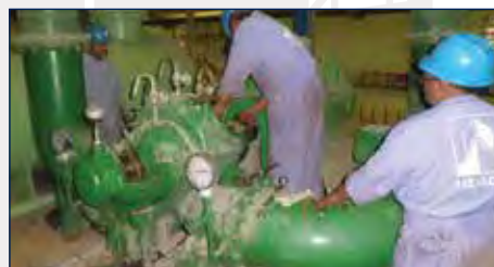
Maintenance of Cooling Water Pump - MEW Shuaiba South Power Station
