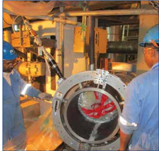
On-site Cold Cutting Services - MEW Doha West Power Station
